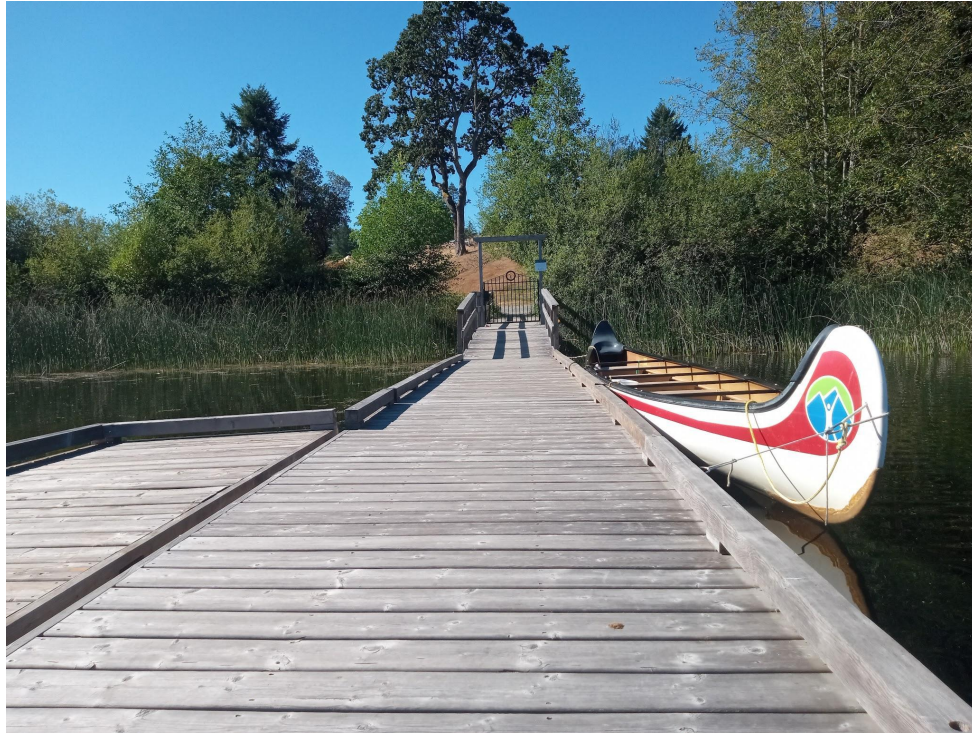
Figure 5. Looking south towards the entrance to the dock.
